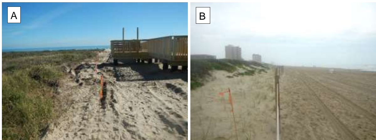
Figure 38. (A) Photo from January 2018 looking seaward from the retaining wall of the impacts to the dune system at SPI02 after construction of the dune crossover. (B) Newly planted vegetation and protective fencing on the seaward dune face at SPI02 in April 2024.
