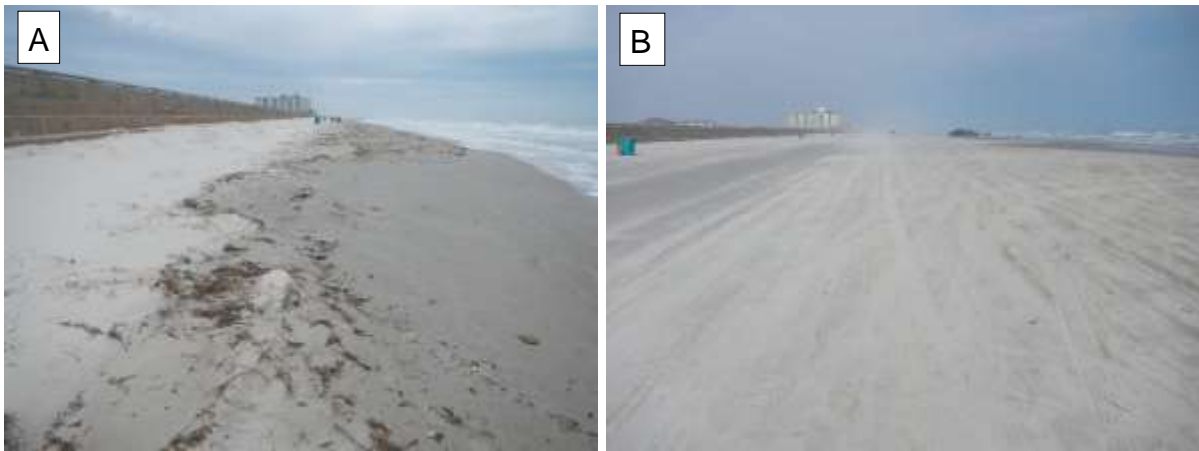
Figure 35. Change in beach width at NPC06 at the southern end of the North Padre Island seawall (A) in January 2022 before a beach nourishment project and (B) February 2024 after the project was completed.
