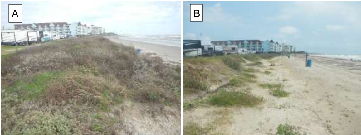
Figure 22. Photos looking northeast at the Dellanera RV Park adjacent the Galveston seawall from (A) January 2020 and (B) April 2024 showing erosion of the dune restoration project.
