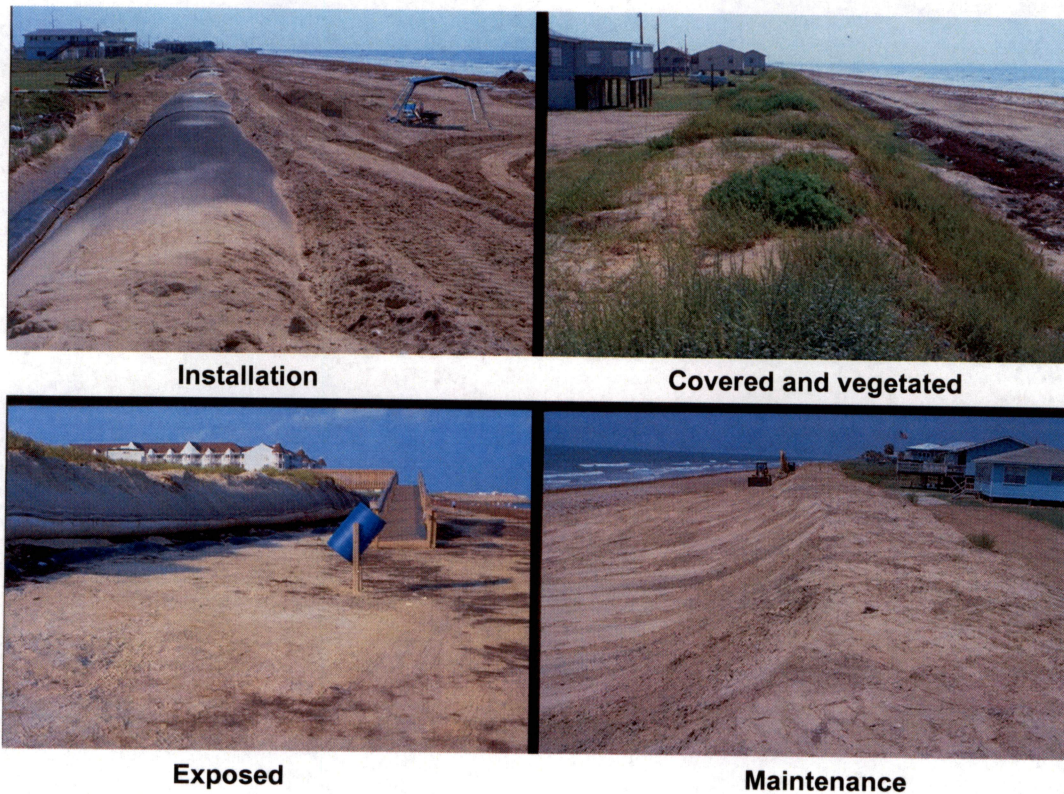
Figure 2. Geotextile tube stages.
