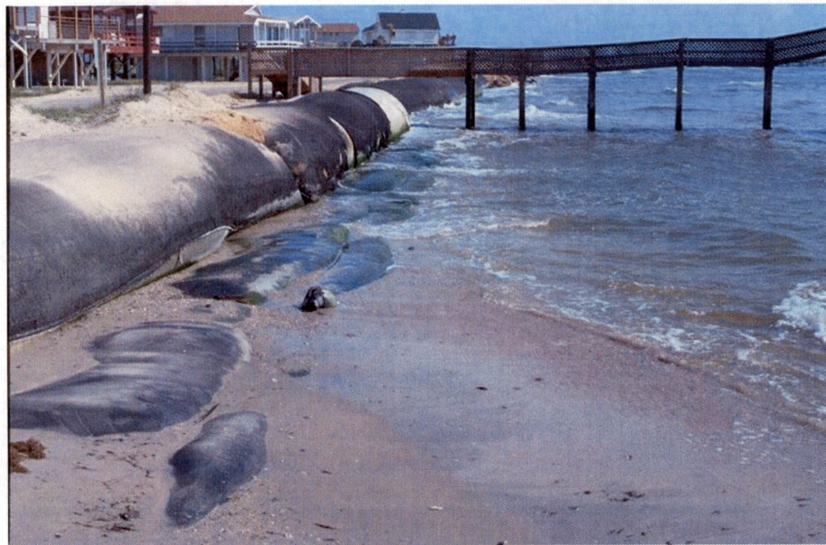
Figure 25. Treasure Island middle geotextile tube on July 19, 2001. Except for a short piece in the foreground this section was completely destroyed in November 2001. Note exposed scour apron and damaged UV shroud. Tube has begun to loose its shape and slump seaward in places.
