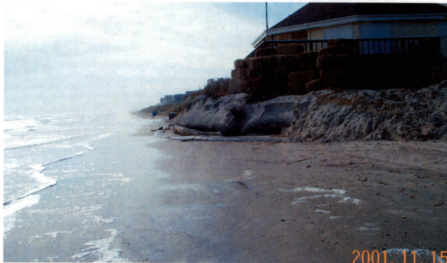
Figure 28. Pirates Beach geotextile tube on November 15, 2001. The tube at this location was routed seaward of the house causing a particularly narrow beach and difficulty in maintaining a sand cover. Water level was about 1 ft (0.3 m) above mean higher high water.
