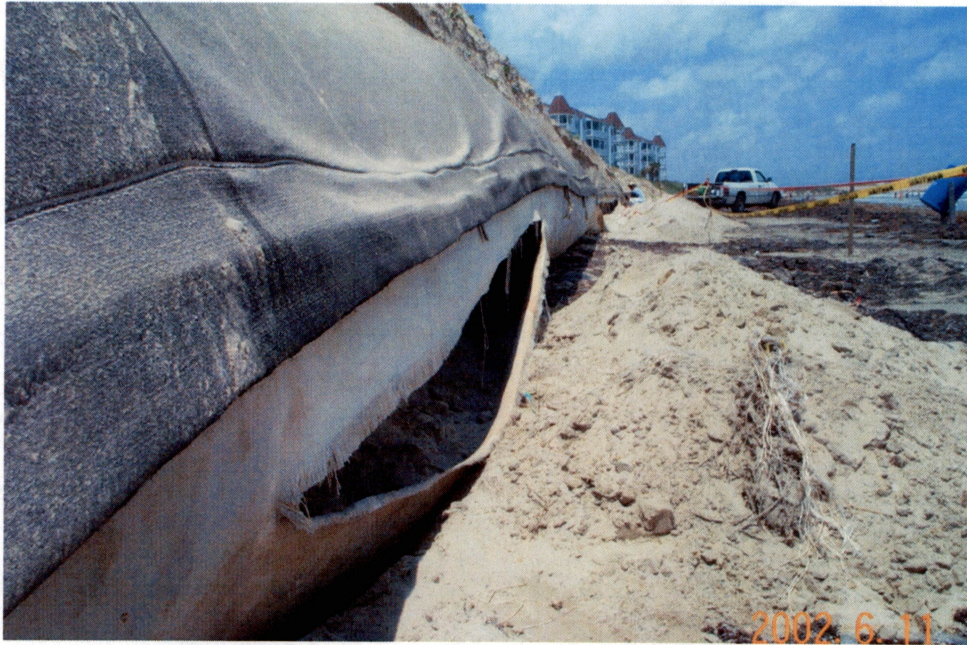
Figure 22. Tear in Dellanera geotextile tube on June 11, 2002. Some have speculated that this hole was the result of vandalism. It has since been patched
