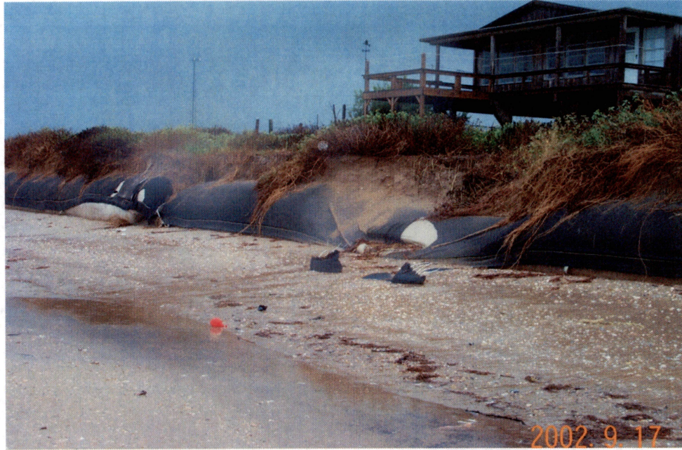
Figure 24. Collapsed geotextile tube section along west end of Gilchrist West project on September 17, 2002 after Tropical Storm Fay.
