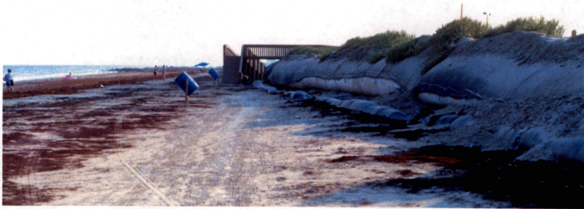
Figure 7. Example of fully exposed geotextile tube front and scour apron at the Dellanera project on Galveston Island, July 18, 2001.
