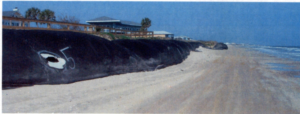
Figure 23. Slumped and collapsed geotextile tube with patched hole near east end of Gilchrist West project (in Caplen) on March 10, 2003. Note completely collapsed section in distance where tube turns seaward.
