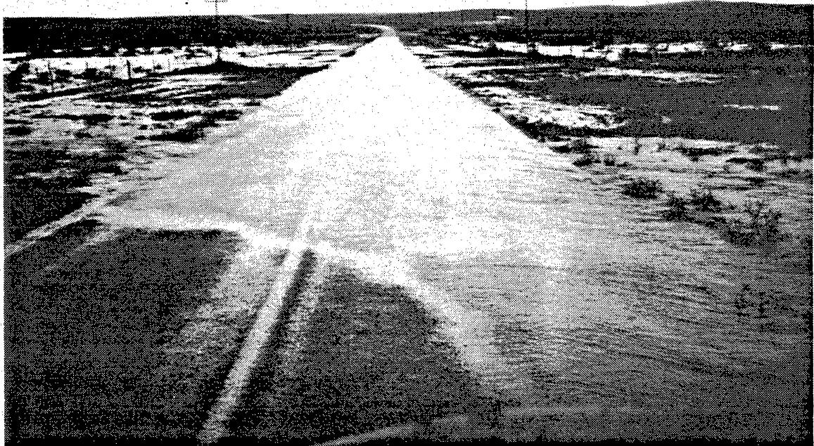
Figure 3. Photograph of flooding at Antelope Draw where it crosses Ranch-to-Market Road 1111. The flood created a body of water 2 ft (0.6 m) deep and as much 200 to 300 ft (60 to 91 m) across. Duration of flooding was very brief, and the highway became passable almost as soon as rainfall terminated.
