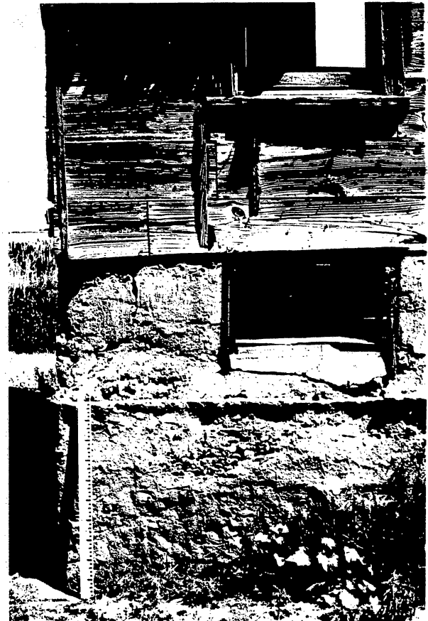
Figure 173. (a) Abandoned homestead, located 5.2 km north of Needmore, in Bailey County, Texas, along State Highway 214. The house was constructed in 1928, abandoned in 1940, and exhibits a maximum of 1.02 m of deflation around its concrete foundation. (b) Detail of exposed foundation, the lower half of which retains impressions of trowel marks and root traces. The concrete forming this part of the foundation was poured against the wall of a shallow excavation. The original ground level is indicated by the rim of concrete at the top of the 1-m scale bar.
