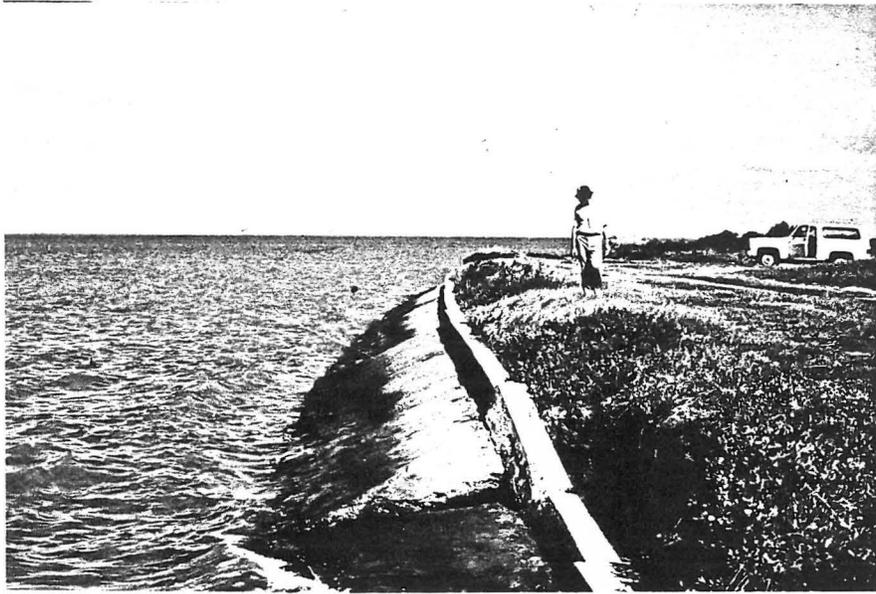
Figure 5-8. Cement bulkhead along the eastern shore of San Antonio Bay south of Seadrift.
