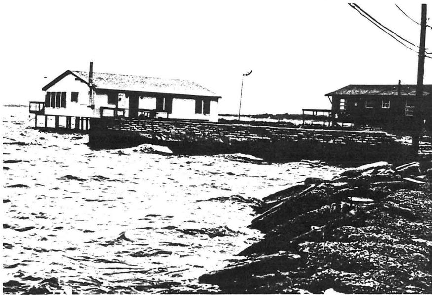
Figure 4-11. Riprap and bulkheads protecting Seabrook, Galveston Bay.
