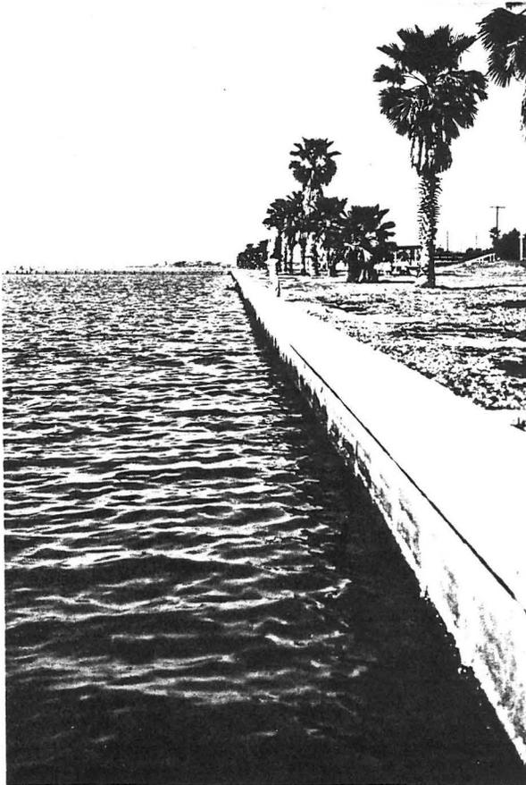
Figure 5-17. Cement bulkhead constructed in 1961 along the shoreline of San Antonio Bay at Seadrift.
