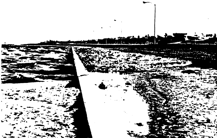
Figure 10. Low concrete bulkheads backed by consolidated riprap and graded fill at Cole Park, southern Corpus Christi Bay.
