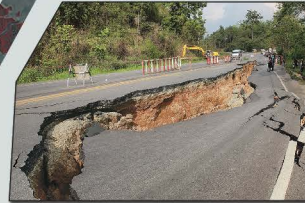
Crack of asphalt road after earthquake. ( www.123rf.com )
