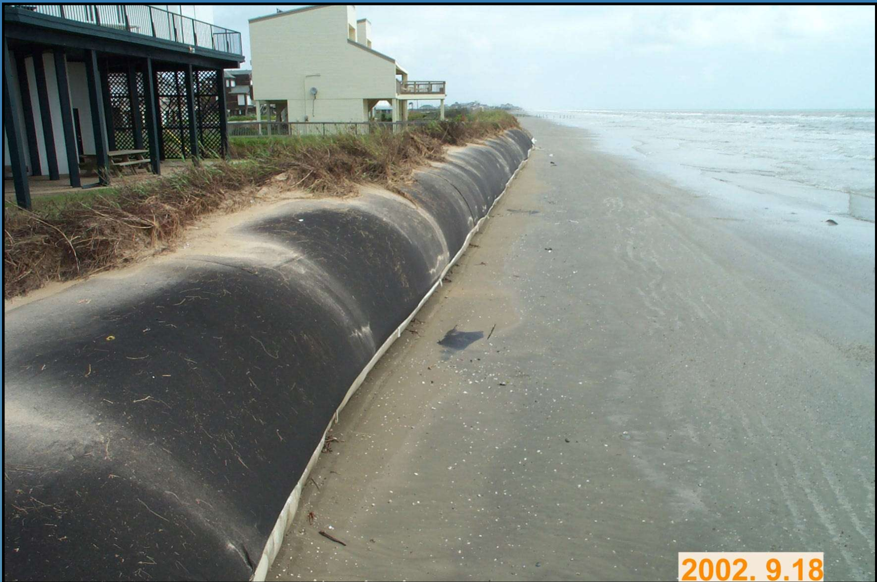
Pirates Beach geotube at GAL02 profile location on September 18, 2002. This geotube was uncovered following Tropical Storm Fay. Note lack of coppice-mound subenvironment when compared with the GLO06 profile location.
