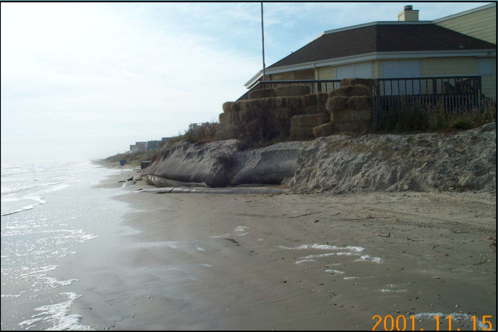
Pirates Beach geotube on November 15, 2001. Geotube at this location was routed seaward of the house, creating a particularly narrow beach and difficulty in maintaining a sand cover on the geotube. Water level was about 2.0 ft (0.61 m) above mean sea level.
