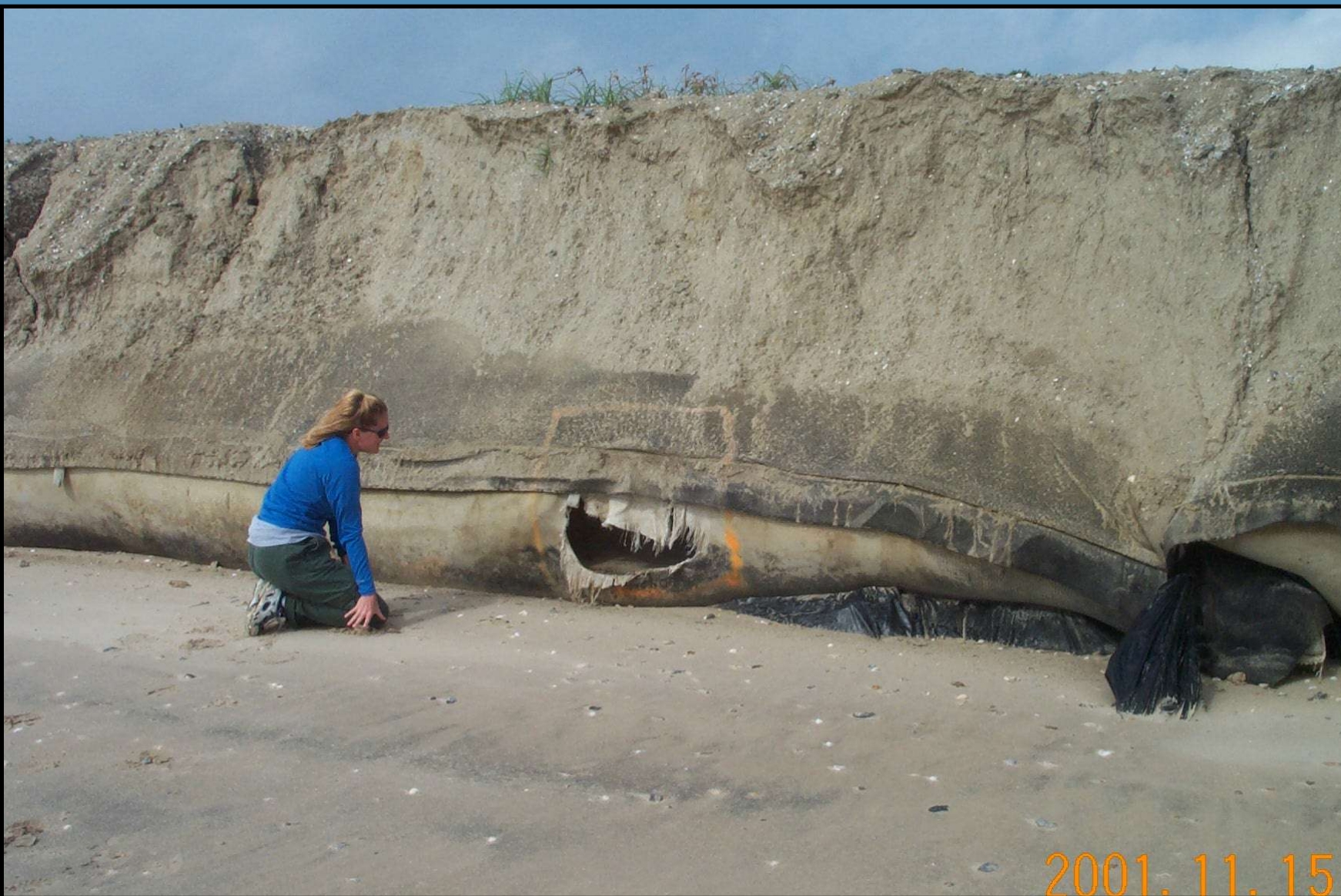
Puncture in Gilchrist West geotube on November 15, 2001.
