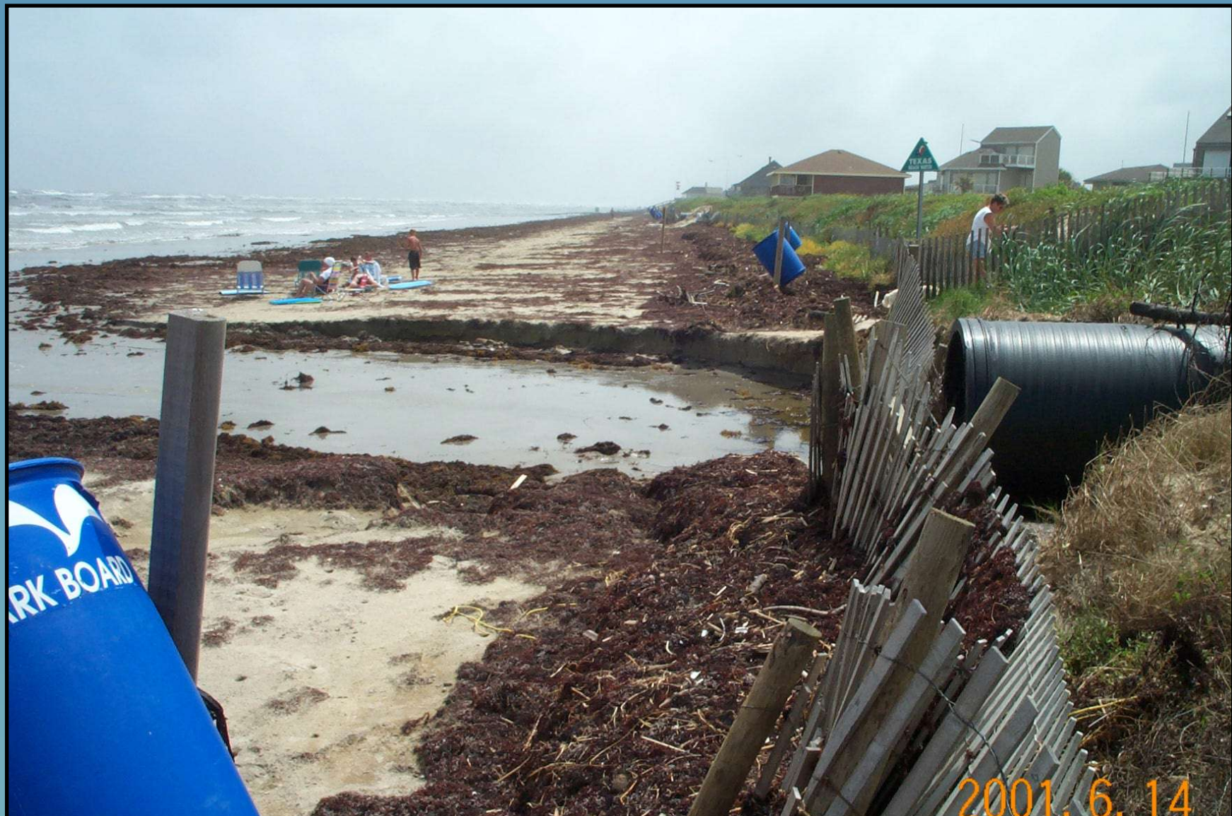
Pirates Beach geotube project on June 14, 2001, after Tropical Storm Allison. Rainfall runoff from Allison flowed through the black street-drainage pipe beneath the geotube on the right and eroded this channel in the beach.
