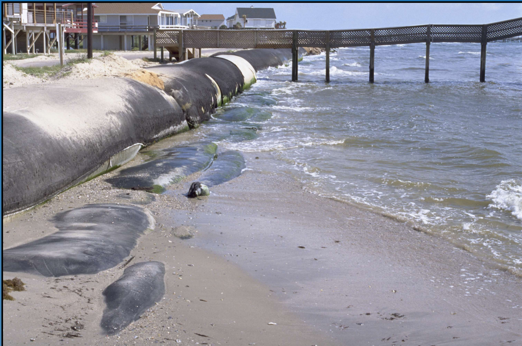
Exposed geotube on July 19, 2001 in the Treasure Island project. This section was destroyed four months later in November, 2001 during slightly elevated (1 ft.) water level and wave conditions. Note exposed scour apron and damaged UV shroud.
