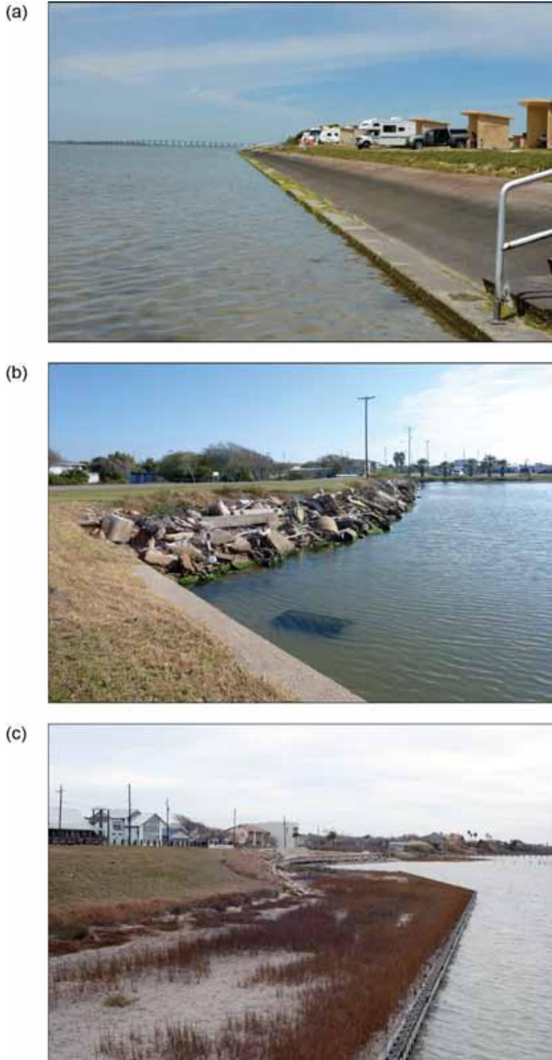
Figure 19. Photographs of shorelines protected by (a) a low seawall at Goose Island State Park on the northern shore of Aransas Bay, (b) riprap and a low concrete bulkhead at Seadrift on the northern shore of San Antonio Bay, and (c) a low bulkhead and vegetation at Bayside on the southwestern shore of Copano Bay.
