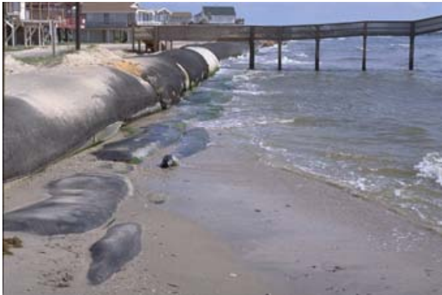
Figure 25. Treasure Island middle geotextile tube on July 19, 2001. Except for a short piece in the foreground this section was completely destroyed in November 2001. Note exposed scour apron and damaged UV shroud. Tube has begun to lose its shape and slump seaward in places.
