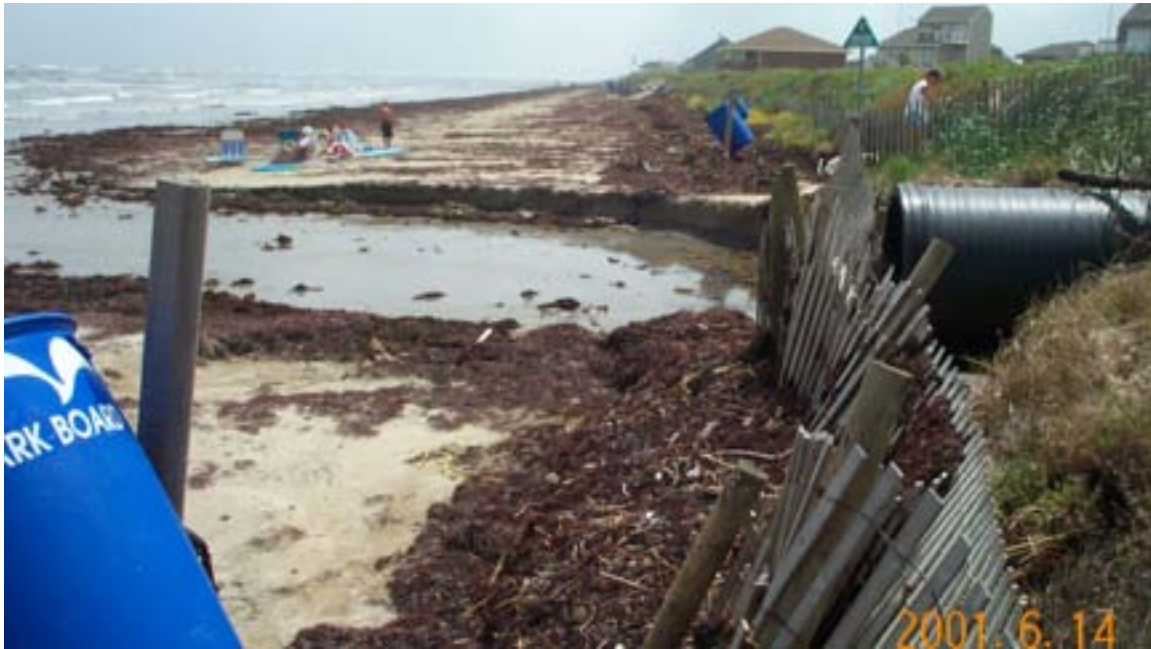
Figure 30. Pirates Beach geotextile tube project on June 14, 2001 after Tropical Storm Allison. Rainfall runoff from Allison flowed through the black street drainage pipe beneath the tube on the right and eroded this channel in the beach.
