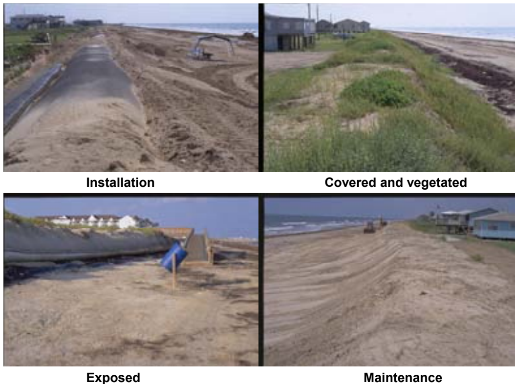
Figure 2. Geotextile tube stages.
