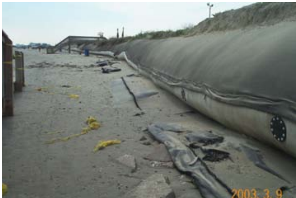
Figure 21. Seaward scour apron exposed and damaged and patched holes in Dellanera geotextile tube on March 9, 2003.
