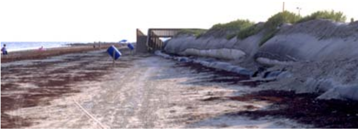
Figure 7. Example of fully exposed geotextile tube front and scour apron at the Dellanera project on Galveston Island, July 18, 2001.
