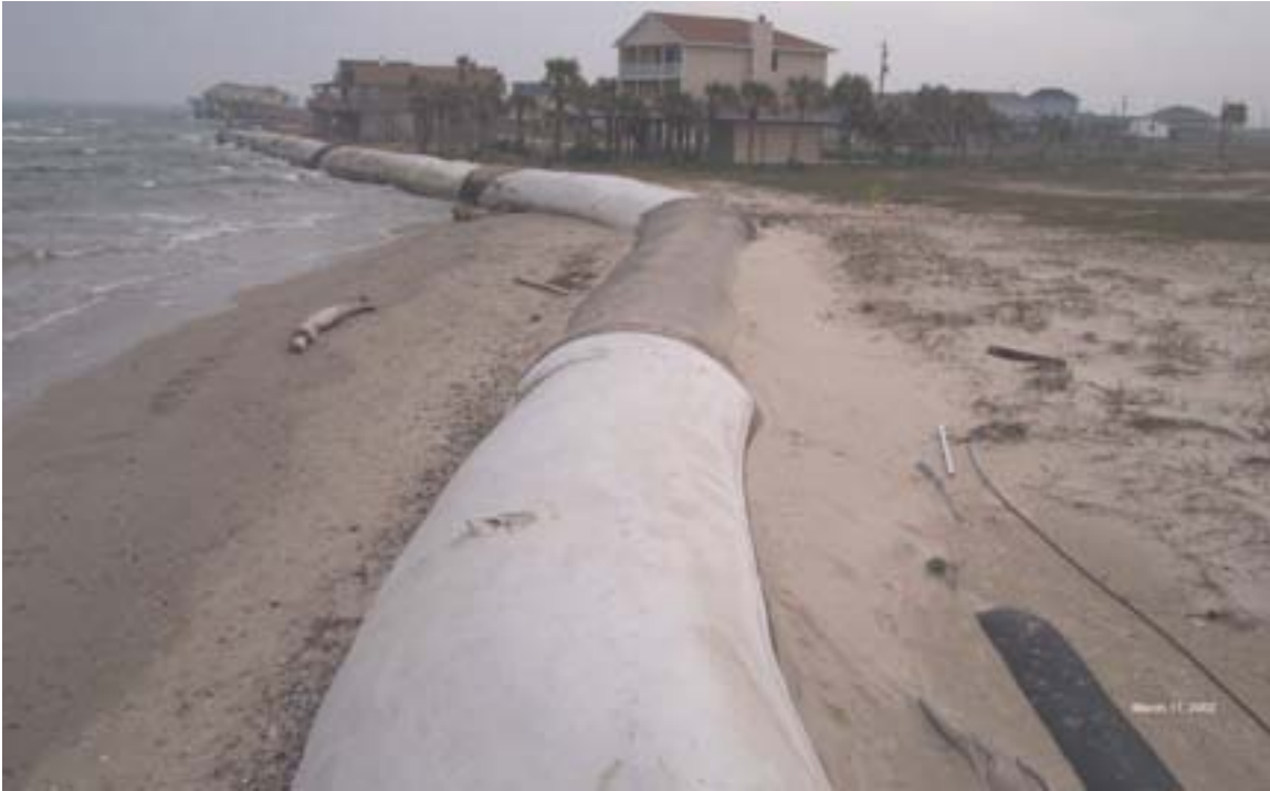
Figure 26. Treasure Island north geotextile tube on March 11, 2003. The UV shroud was almost completely destroyed and erosion had occurred behind the tube with some wind-blown sand deposited between the landward side of the tube and the erosional scarp.
