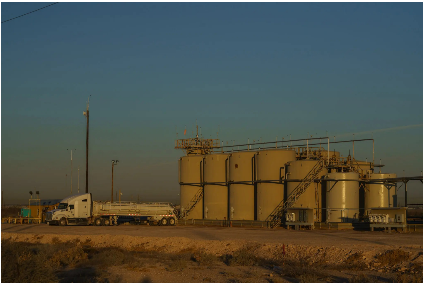
A saltwater disposal site. Some of that water that is a byproduct of hydraulic fracking is reused, but most of it is injected back under the ground. Paul Ratje for The New York Times
