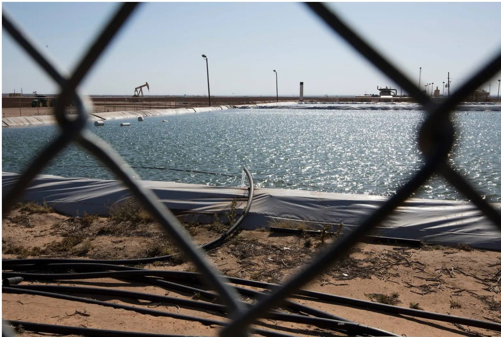
A fracking water retention pond near Big Spring. Wells in the Permian Basin generate six times more water than oil, and companies must dispose of the water through injection wells or other means. 📷 Marjorie Kamys Cotera for The Texas Tribune
