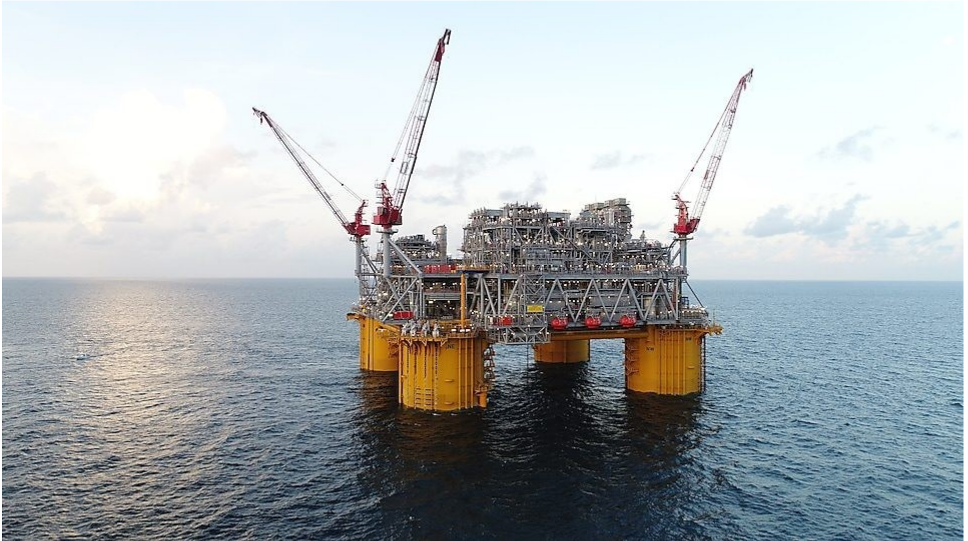
The Appomattox oil platform in the Gulf of Mexico. Source: Shell
