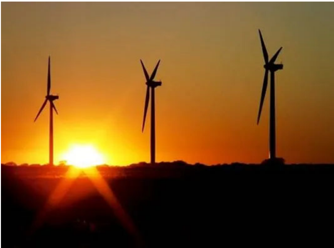
The Pattern Energy Group, a San Francisco company, is building a 118-tower wind farm in Kenedy County. (Photo: Contributed photo)
