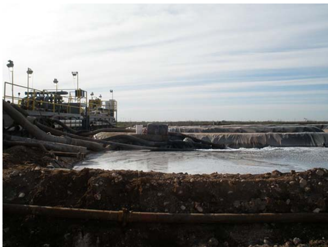
Hannah Hamilton | USGS A fluid impoundment containing produced waters at a hydraulic fracturing drilling operation in the Permian Basin of West Texas.
