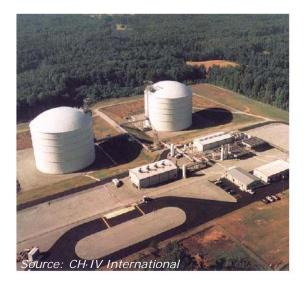
Perhaps most visible type of LNG facilities is *baseload LNG receiving and regasification facilities*. These facilities consist of marine terminals for LNG ships (1), LNG receiving and storage facilities (2), and vaporizing facilities and supporting utilities (3). Figure 8 provides a layout for typical onshore LNG baseload receiving facilities.
