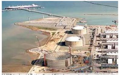
Figure 17. Double Containment Tanks
