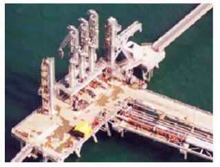
Figure 21. LNG Jetty with Unloading Arms - ALNG
