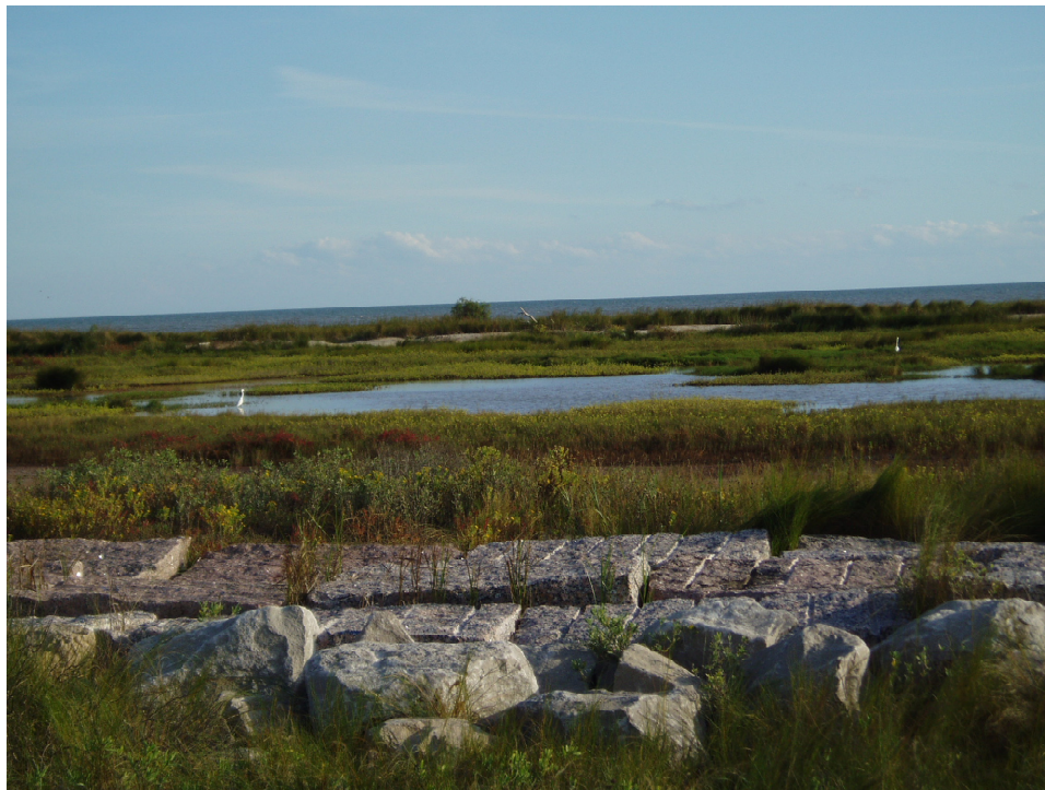
Figure 22. Top of shoreline protection feature constructed to protect the GIWW between Caney Creek and Cedar Lakes. View is gulfward.
