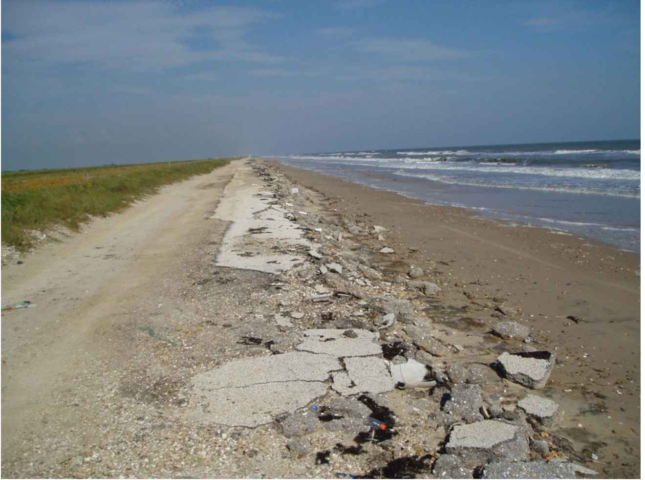
Figure 47. Evidence of Gulf shoreline erosion along the strandplain-chenier system. Photo, taken in October 2006, shows remnants of Highway 87 approximately 6.5 km northeast of High Island.
