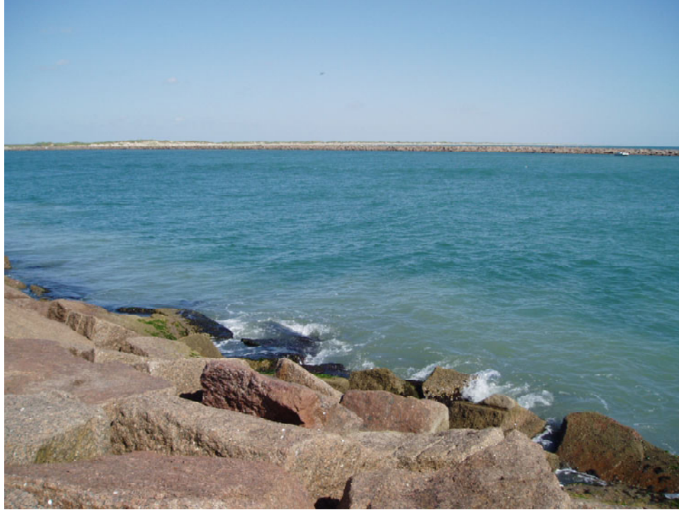
Figure 15. Rip rap along jetties at Mansfield Channel. These features were mapped as M2RS2Pr (Marine intertidal rocky shore, rubble, irregularly flooded, artificial).
