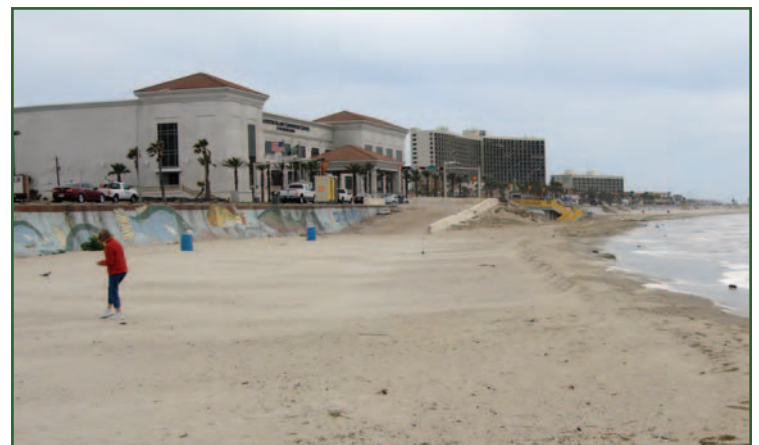
The Galveston Seawall after restoration.
