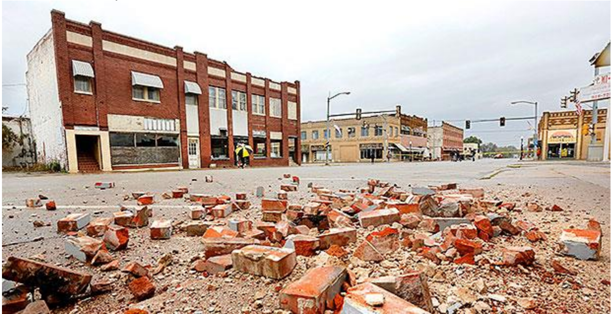
Damage in Cushing, Okla., which was struck with a magnitude 5 earthquake on Nov. 6 last year. Photo by Jim Beckel, courtesy of AP Images.
