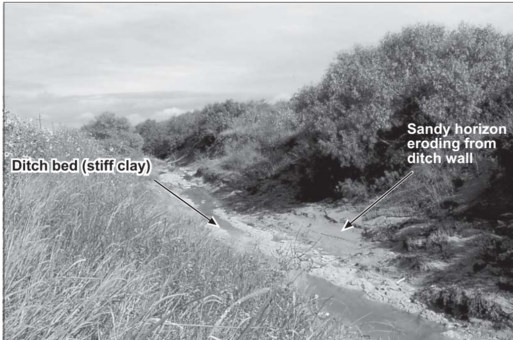
Figure 9. Drainage ditch along Nueces County Road 18 near Driscoll. A relatively sandy horizon is eroding from the ditch wall above stiff clay that forms the bed of the ditch. Both units are within the Pleistocene Beaumont Formation.
