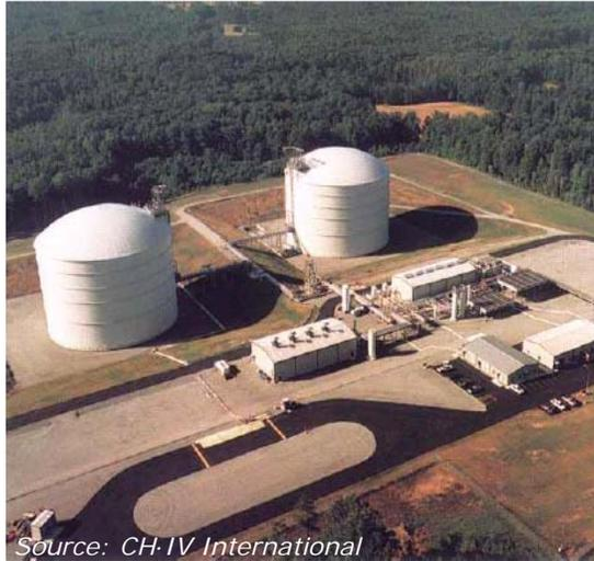
Perhaps most visible type of LNG facilities is *baseload LNG receiving and re-gasification facilities*. These facilities consist of marine terminals for LNG ships (1), LNG receiving and storage facilities (2), and vaporizing facilities and supporting utilities (3). Figure 8 provides a layout for typical onshore LNG baseload receiving facilities.
