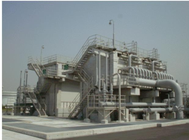
Shell and tube heat exchangers can also use seawater but in this case the heat exchange takes place with the LNG inside tubes and seawater flowing around the tubes inside a shell. This is also a proven technology with slightly higher process intensity due to the controlled fluid flow fields in the shell tube configuration. However, due to the probability of a tube rupture, there is the added reliance on a safety valve in the shell in order to avoid increased pressures and explosion risks.
