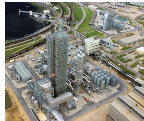
The Petra Nova carbon dioxide extraction facility. The taller structure is the absorption tower. The smaller tower contains the regeneration process. (Photo courtesy of NRG Energy)
