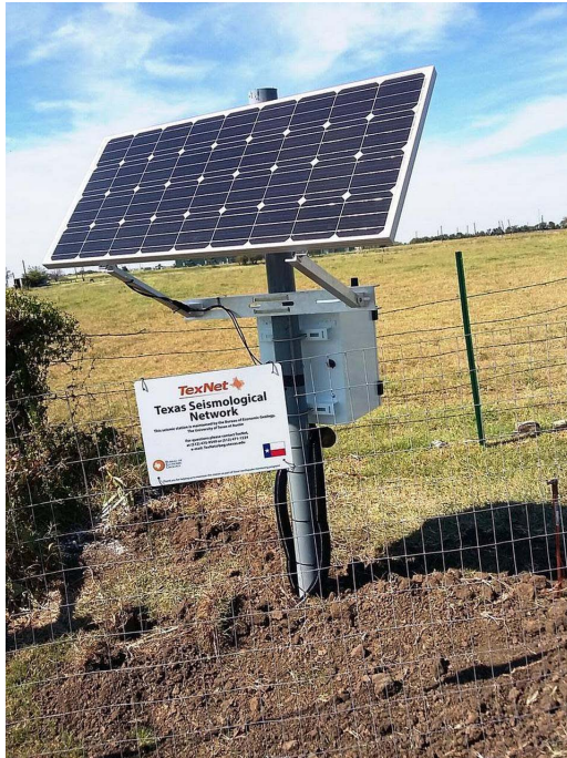
One of the seismometer stations installed by TexNet in the Fort Worth Basin area. Texas Bureau of Economic Geology
