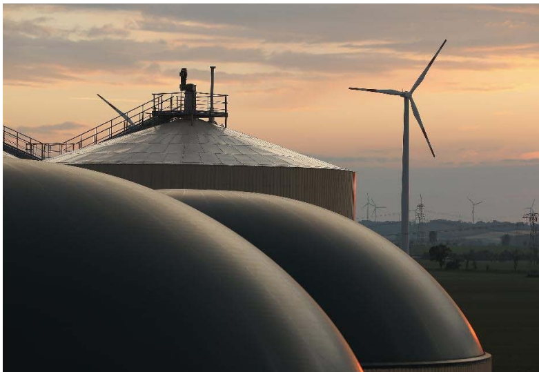
A wind turbine spins behind a new biogas plant in Lower Saxony on June 12, 2012 near Ebendorf, Germany. (Photo by Sean Gallup/Getty Images)
