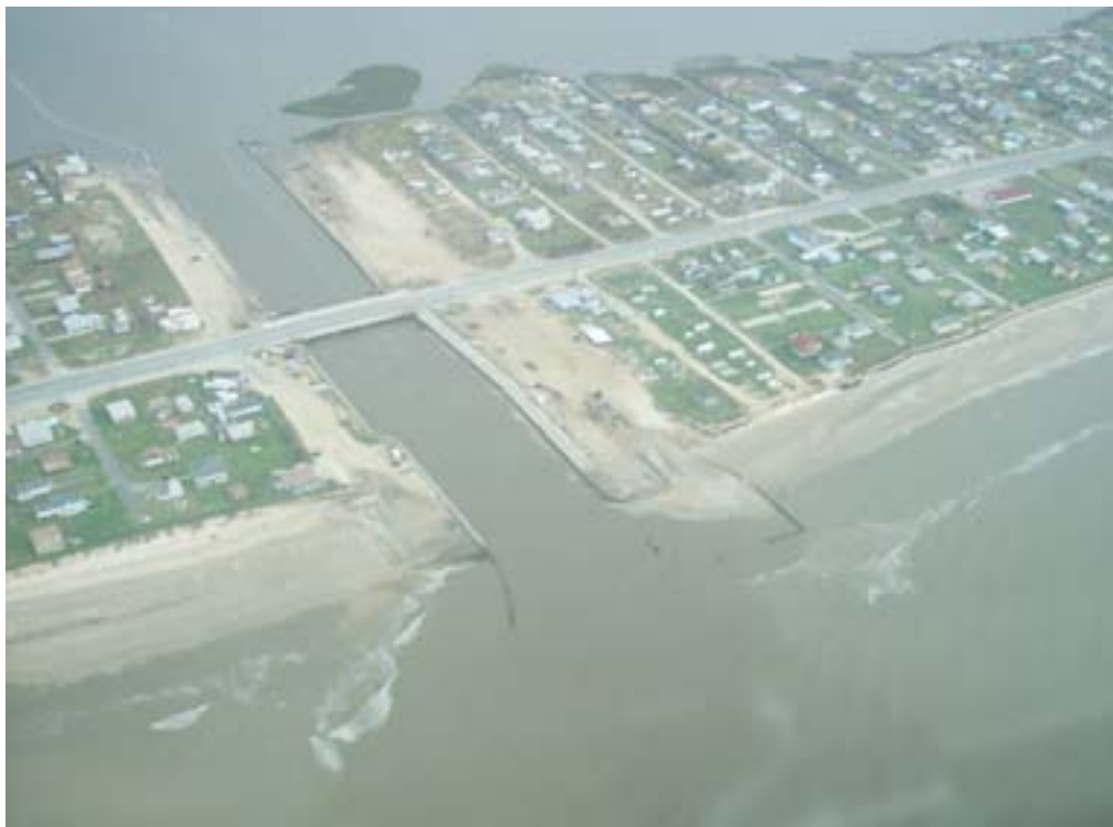
Figure 27. Rollover Pass. Rita caused washover and sand transport through the unpaved parking lots and across highway 87. Geotextile tubes are exposed to the northeast (right) of the pass but not on the southwest side.
