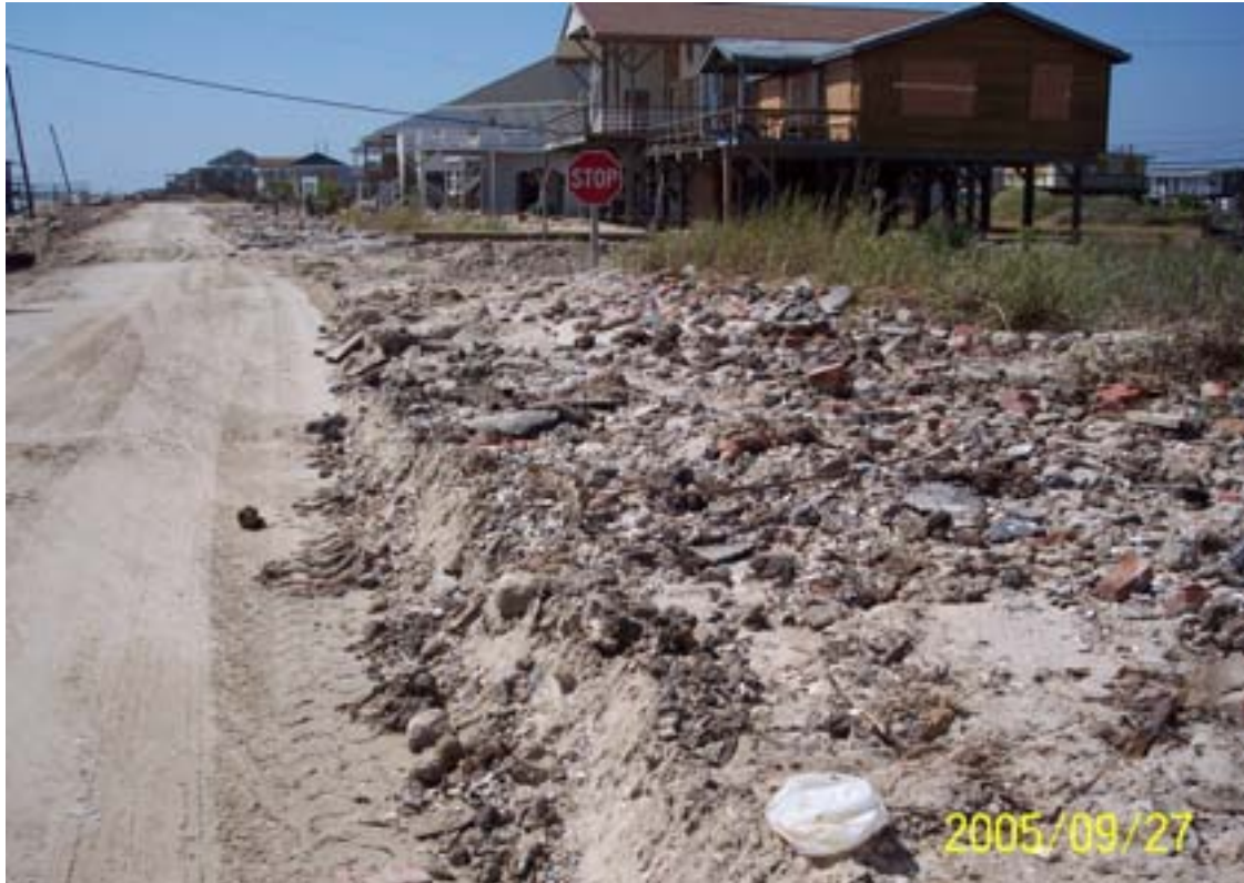
Figure 14. Washover deposition including debris and asphalt pieces transported landward of Beach Drive. Beach Drive has been plowed.
