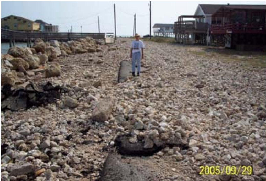
Figure 19. Treasure Island subdivision. Cobbles from shore-protection efforts deposited by Rita's waves on the road.
