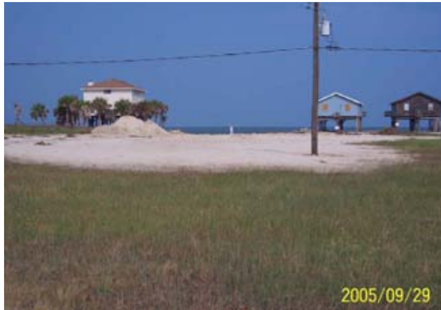
Figure 22. Sandy washover fan deposit in the Treasure Island subdivision. Also note stock piles of sand on left of fan. Piles like these were being placed around Treasure Island.
