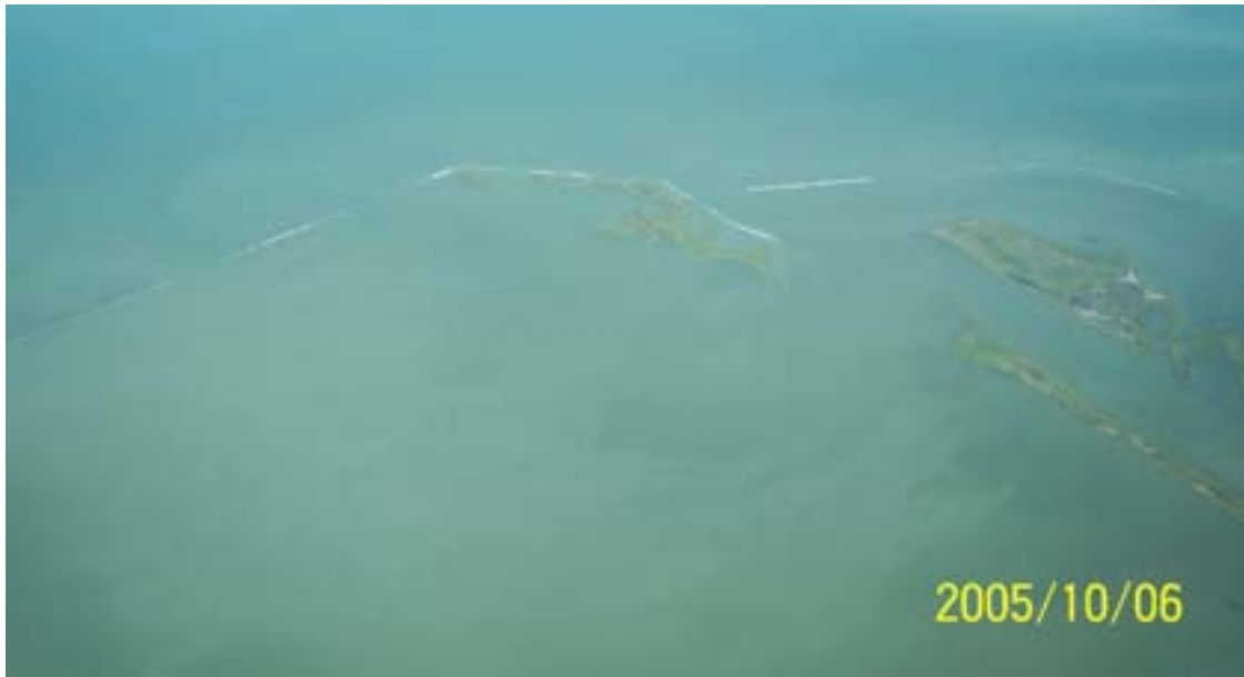
Figure 35. Aerial view of geotextile tubes protecting marsh restoration project in Galveston Island State Park.
