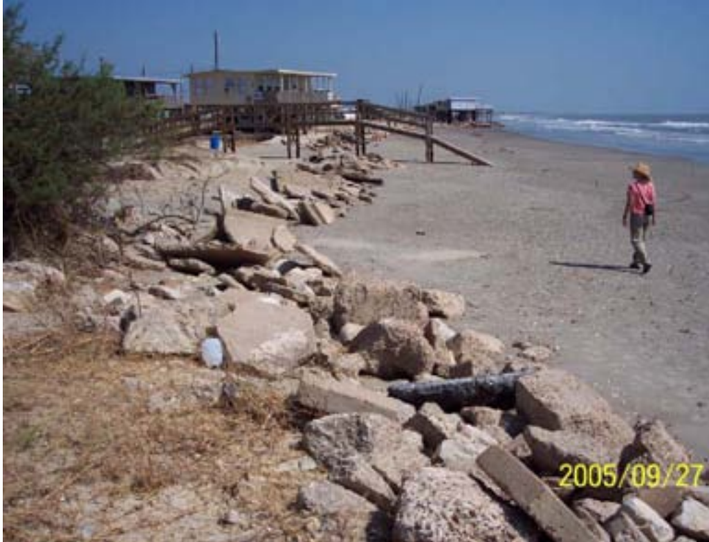
Figure 11. Surfside Beach. Beach eroded and washed over landward of concrete rip rap.
