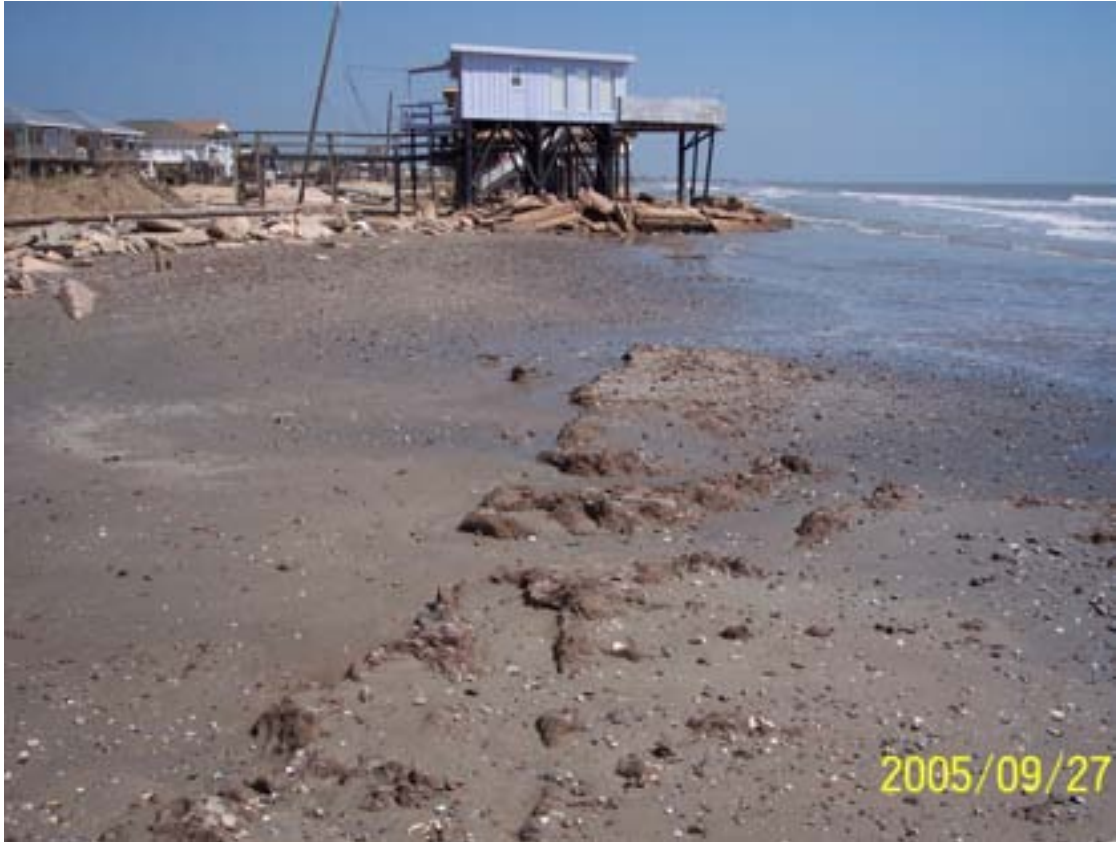
Figure 13. Surfside Beach houses in the surf zone. Layer of Holocene sandy mud exposed in foreground which attests to the erosional state of the beach.
