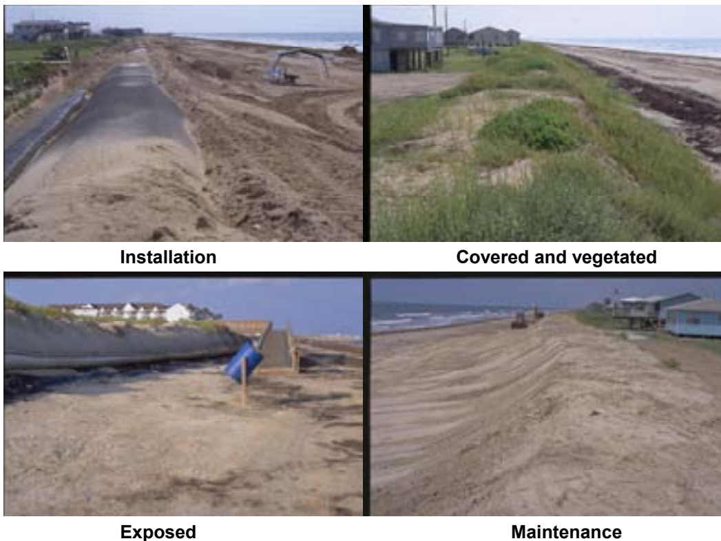
Figure 2. Geotextile tube stages.
