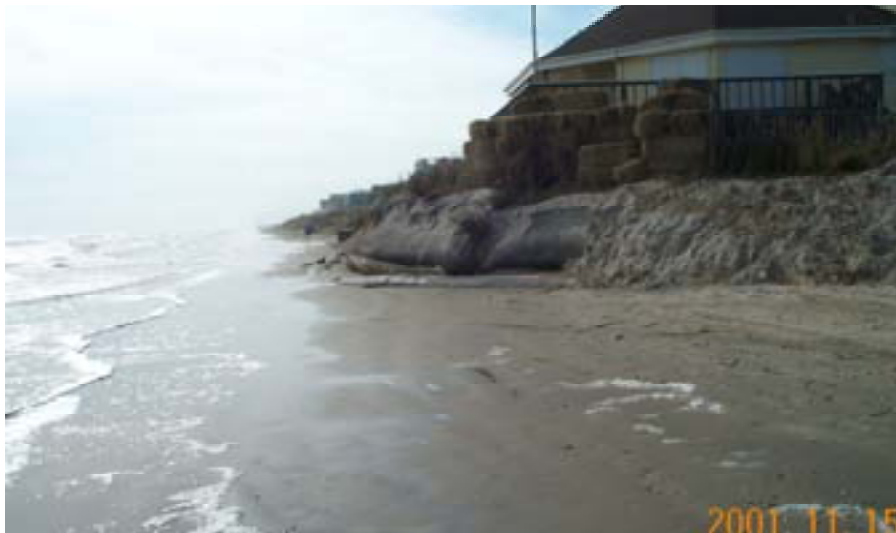
Figure 28. Pirates Beach geotextile tube on November 15, 2001. The tube at this location was routed seaward of the house causing a particularly narrow beach and difficulty in maintaining a sand cover. Water level was about 1 ft (0.3 m) above mean higher high water.
