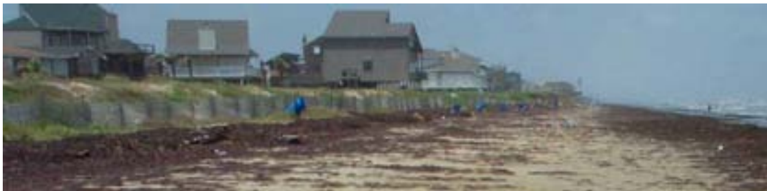
Figure 27. Pirates Beach geotextile tube at GAL01 profile location (see figure 6 for location). This project remained covered and vegetated following Tropical Storm Allison. Note sand fence and lack of coppice mound subenvironment.
