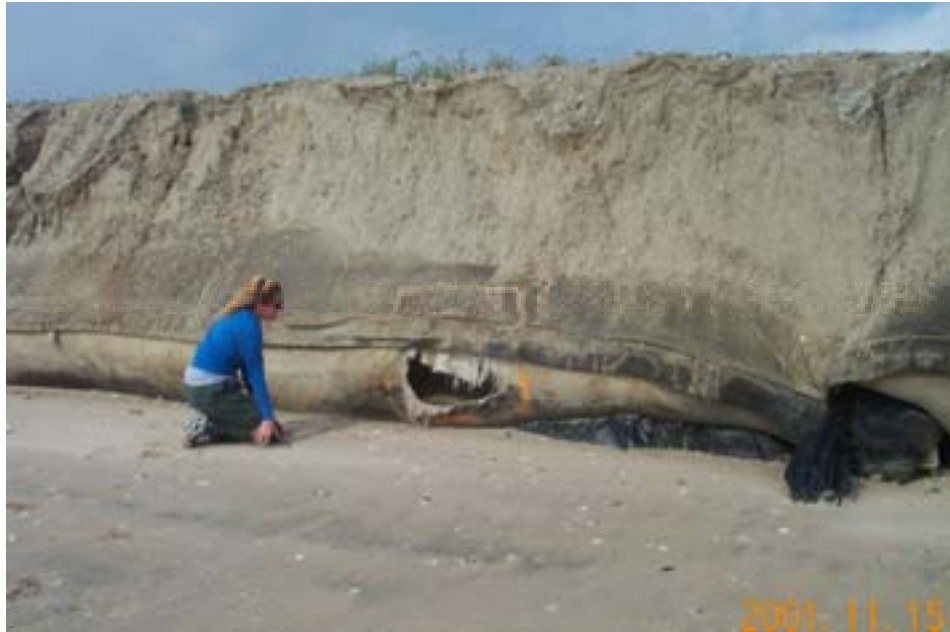
Figure 20. Puncture in Gilchrist West (Caplen area) geotextile tube on November 15, 2001.
