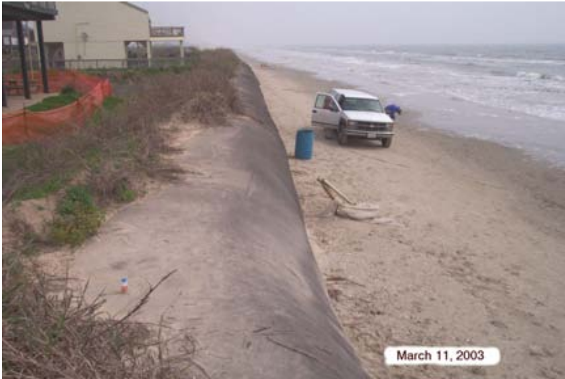
Figure 34. GAL02 beach profile location in the Pirates Beach geotextile tube project on March 11, 2003. There is no coppice mound environment seaward of the tube because the beach is too narrow and too low for vegetation and wind-blown sand to accumulate (see Fig. 6 for location and Fig. 32 for beach profile).
