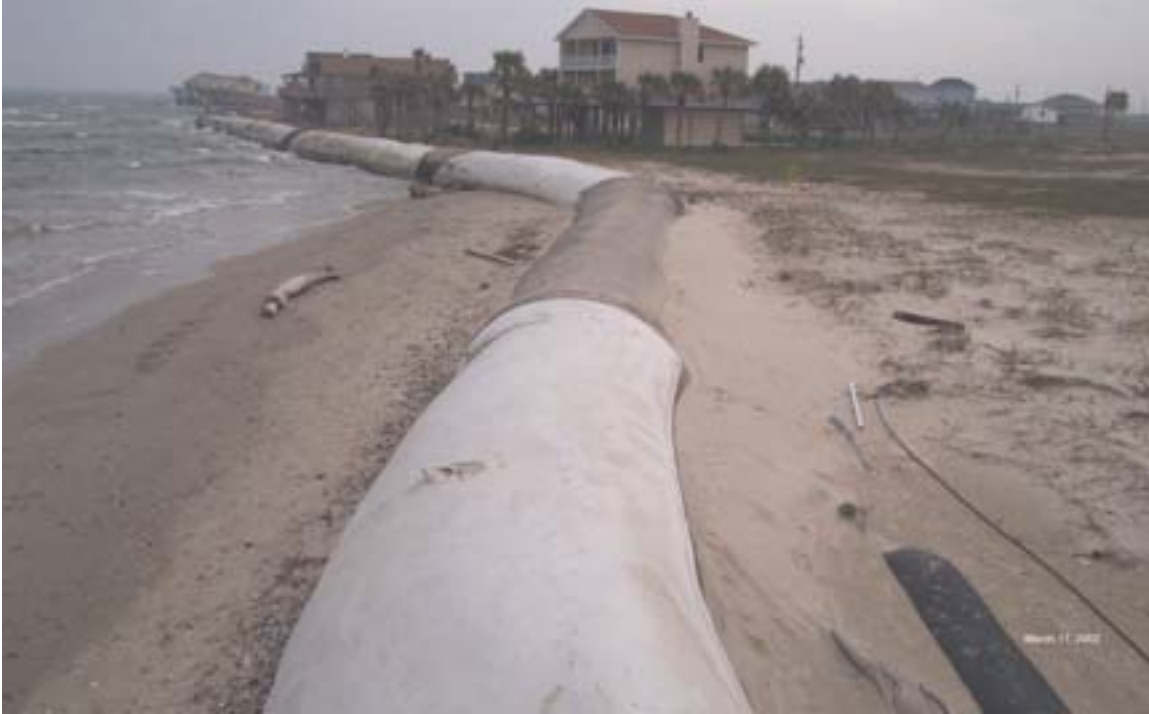
Figure 26. Treasure Island north geotextile tube on March 11, 2003. The UV shroud was almost completely destroyed and erosion had occurred behind the tube with some wind-blown sand deposited between the landward side of the tube and the erosional scarp.
