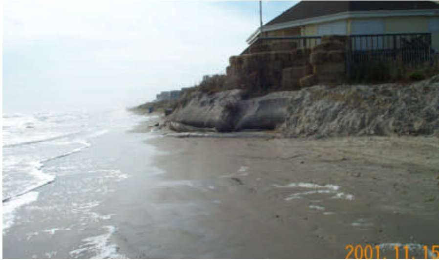
Figure 18. Pirates Beach geotube on November 15, 2001. Geotube at this location was routed seaward of the house causing a particularly narrow beach and difficulty in maintaining a sand cover on the geotube. Water level was about 2.0 ft (0.61 m) above mean sea level.
